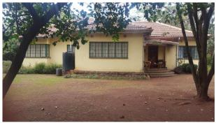
**Roof:** - Pitched roof overlaid with clay bricks and fitted with rainwater gutters and downpipes at the eaves.
