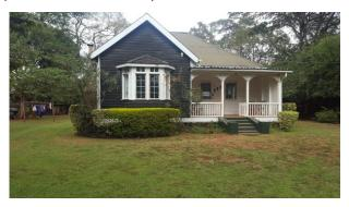
**Roof:** - Pitched roof overlaid with galvanized corrugated iron sheets and fitted with rainwater gutters and downpipes at the eaves.
