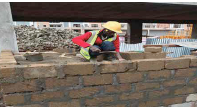
Gatehouse walling ongoing.
