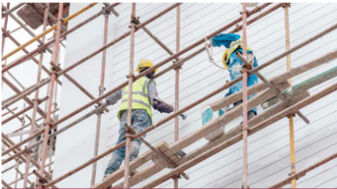
External walls skimming is ongoing.
