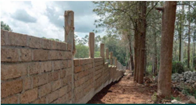
Superstructure walling on the western boundary.
