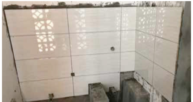
Kitchen yard tile fixing ongoing.
