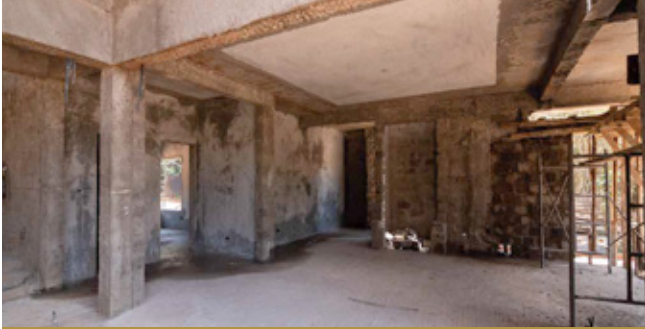
Plaster works at the ground floor area in progress.
