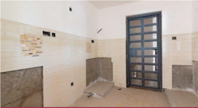
Kitchen yard door installation.
