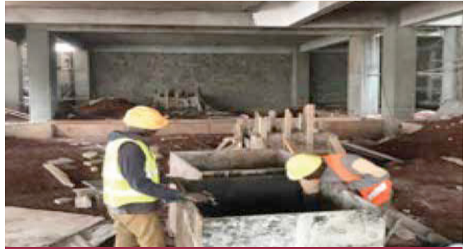
Formwork for sewer manholes ongoing.
