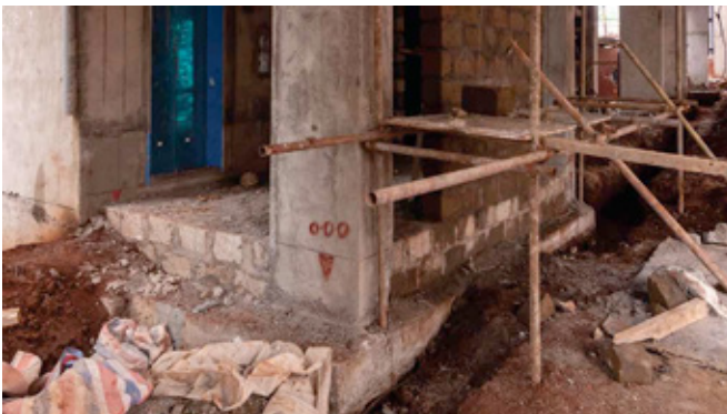
Kitchen trunk line UPVC installation.
