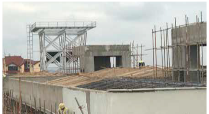
Installation of timber battens ongoing.
