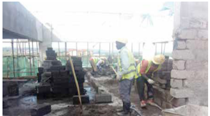
12th Floor masonry walling.
