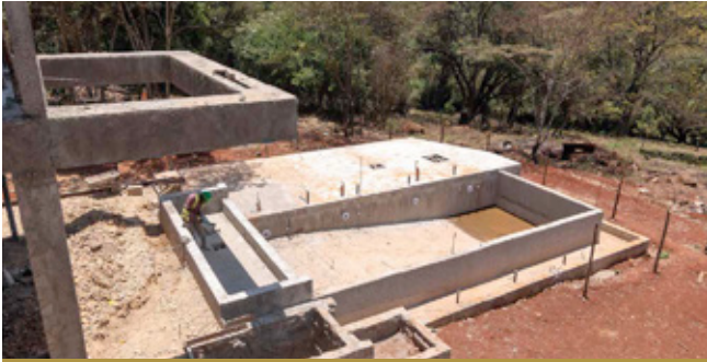
Works at the swimming pool area are ongoing.
