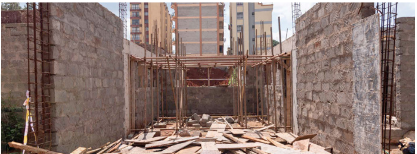
Nursery ground floor walling.
