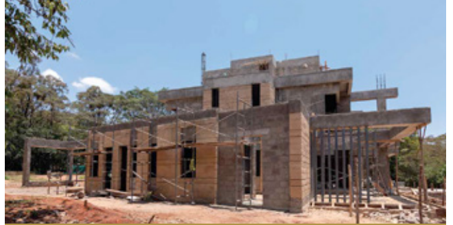
External cladding at the DSQ is complete.
