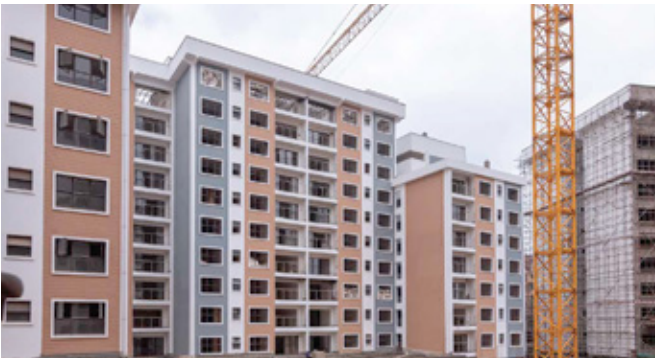
External facade paint is ongoing.
