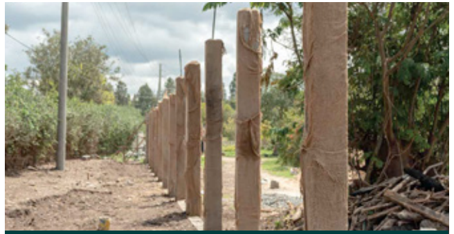
Columns in progress along the road frontage.
