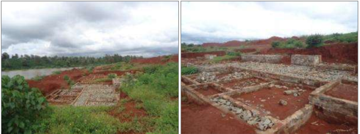
-Views of the units under construction-
