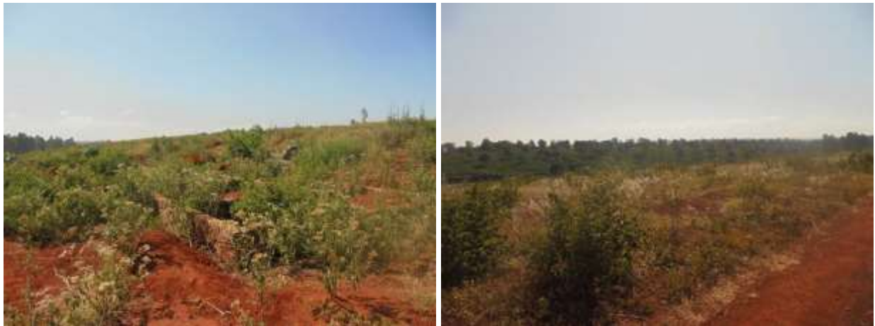
-Views of the units under construction-
