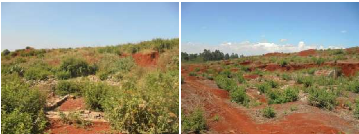
-View of some of the vandalized units on site-
