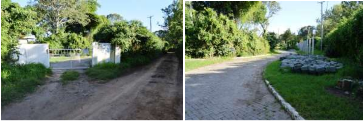
-Views of the Main Gate and Access Road-
